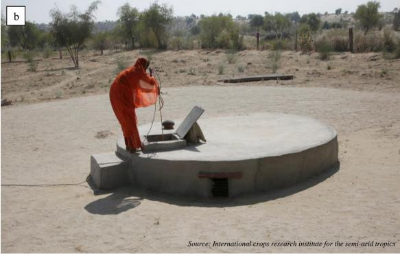
Figure- 1 (a) & (b): KUND system of rain water harvesting
