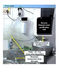
Plate1. Reverse osmosis water purification unit used in select households
